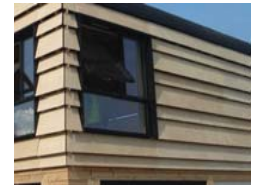
composite & painted timber weatherboard
