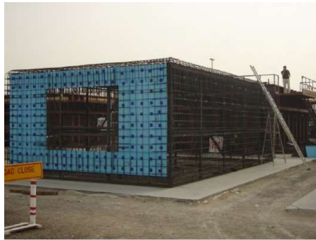
Step 1 – Reinforcing & Insulation
