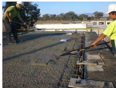
Step 5 – 40MPa Concrete Poured
