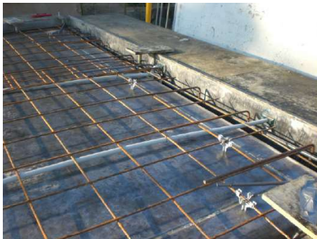
Step 4 – M E P Positioned
