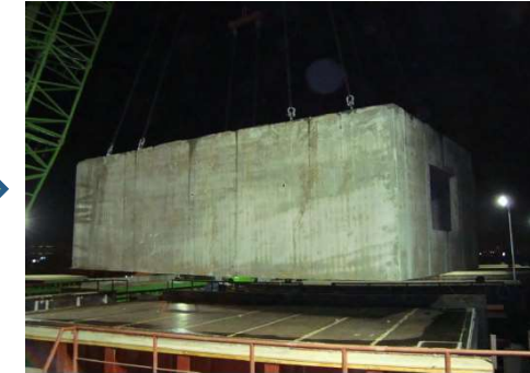
Step 6 – Cured Module Lifted
