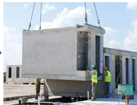
Step 10 – Crane Into Position
